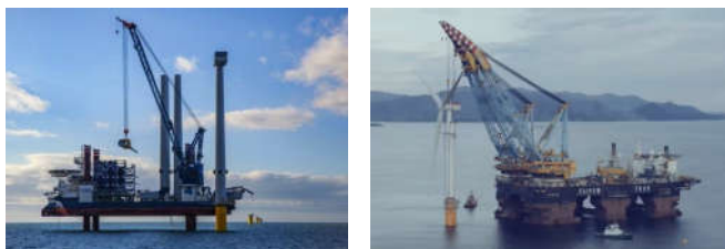
Figure 1: Examples of offshore wind farms during installation (left: First MHI Vestas 8MW wind turbine installed by A2Sea jack-up Sea Installer in Burbo Bank 2 offshore wind farm in UK (Renews, 2017); right: Spar floating wind turbine assembled in Norway by SAIPEM 7000 before towed to Statoil Hywind offshore wind farm in Scotland (Statoil, 2017))
